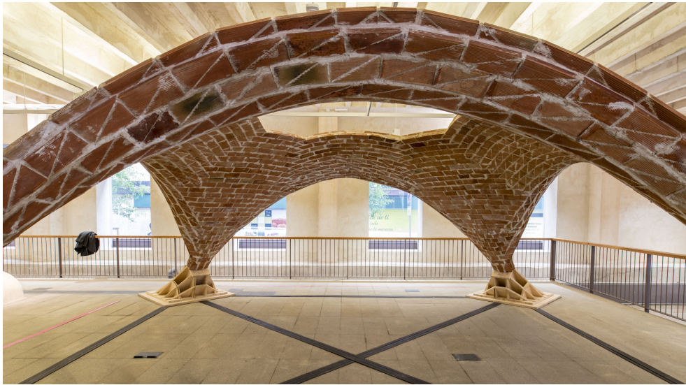
Figure 2: Timbrel vault (SOM and University of Alcalá, 2019)
