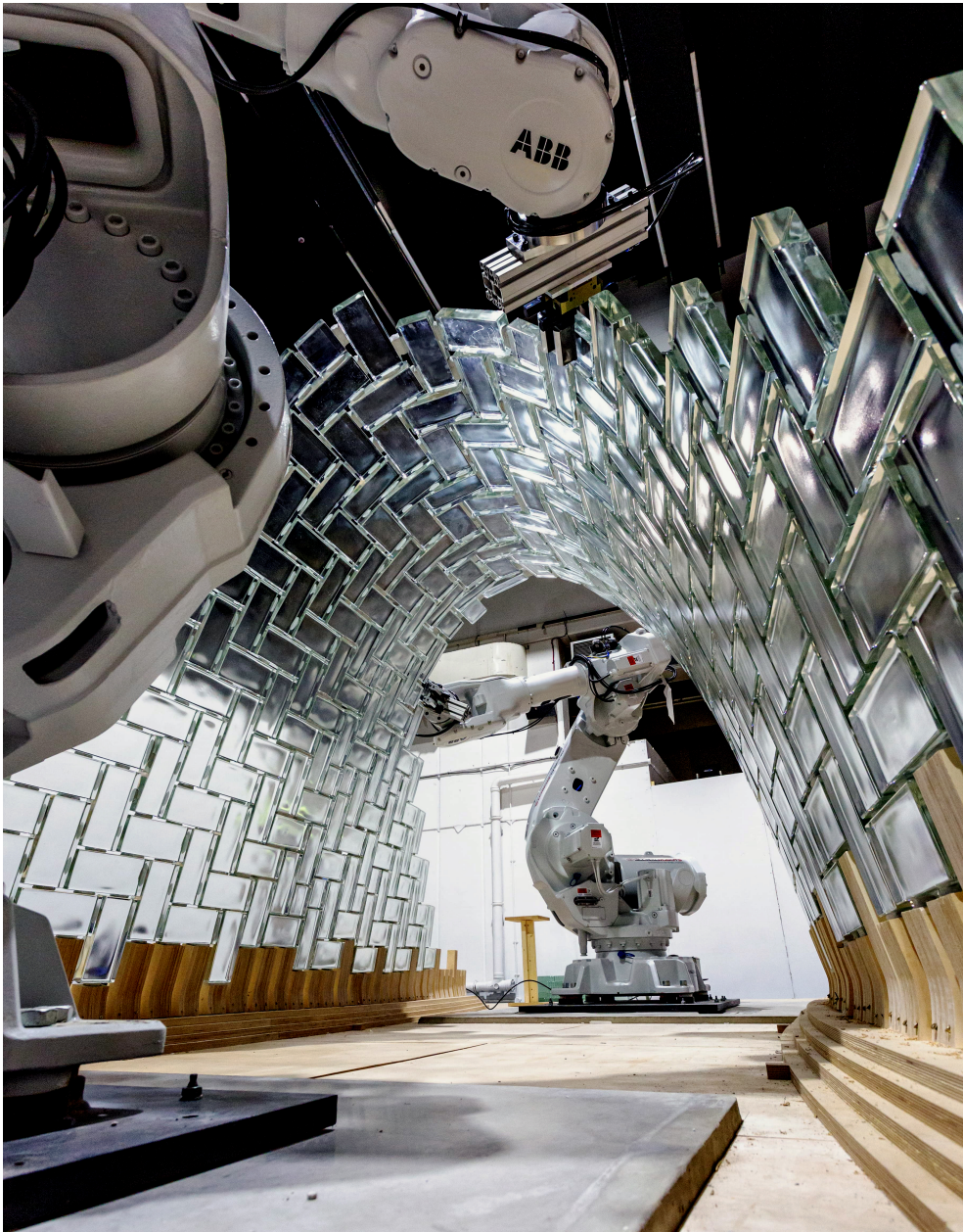
Figure 20: Final constructed vault
