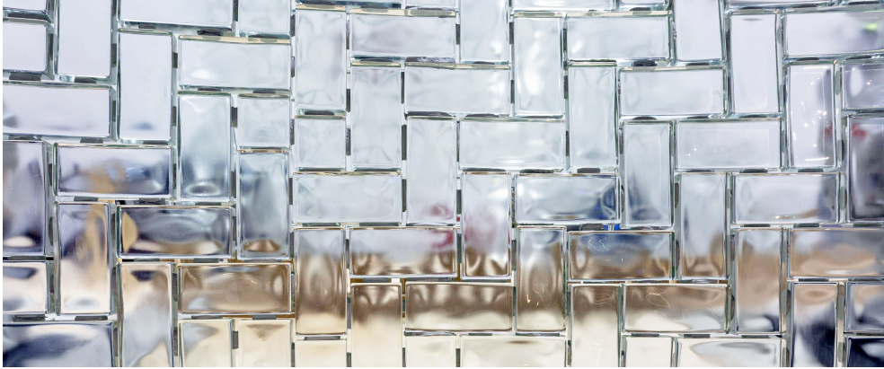
Figure 5: Herringbone tessellation pattern with glass bricks in the constructed vault
