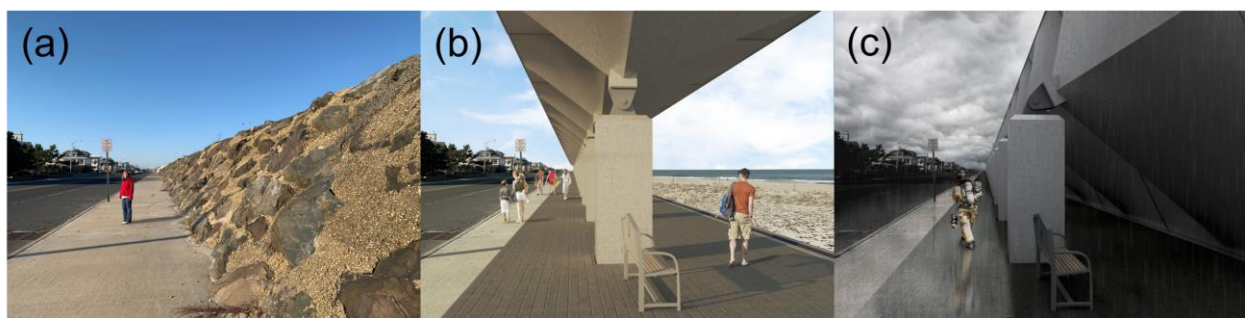
Fig. 1. a) Seawall at Monmouth Beach, NJ; b) Upright Kinetic Umbrellas; c) Tilted Kinetic Umbrellas for coastal defense
